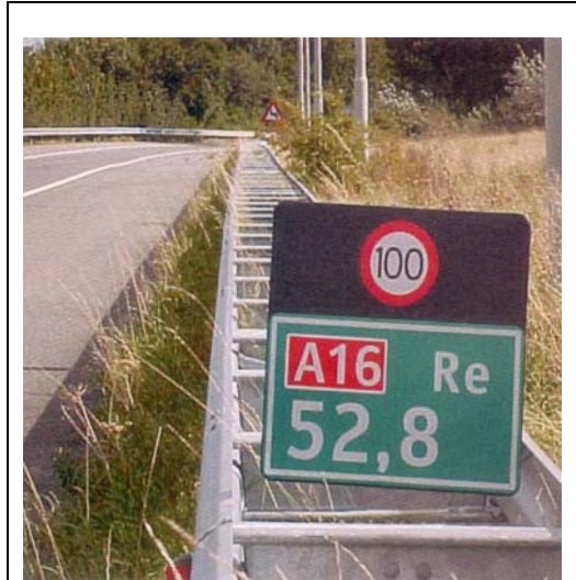
A hectometre post with speed limit reminder at motorways in the Netherlands
